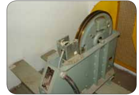
Figure 10: Fingers may get pinched at the moving parts that are left uncovered.
