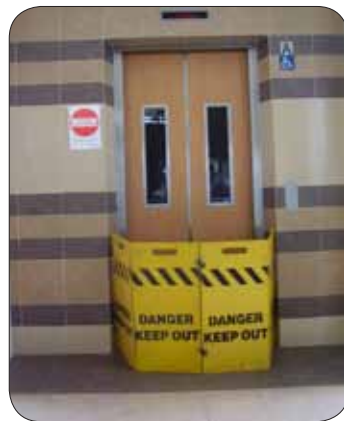
Figure 34: An example of using lift barrier to warn the public of falling hazards.
