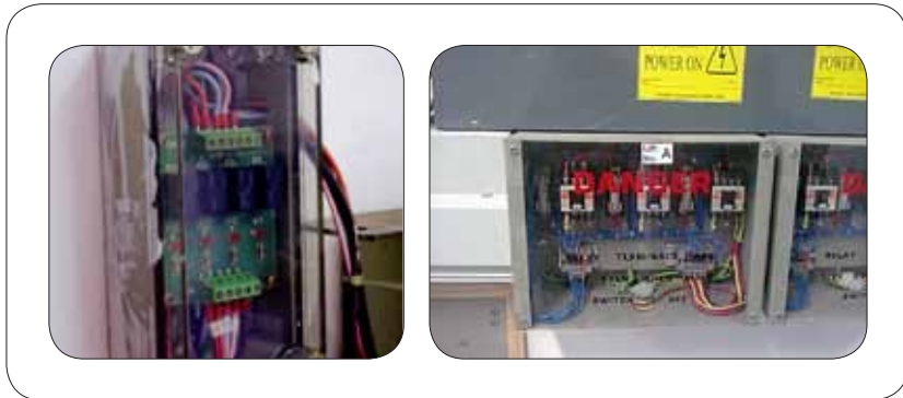
Figure 30: Examples of finger-safe terminal block.
