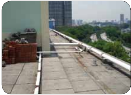
Figure 17: Falling off open sides at the roof or edges of buildings.
