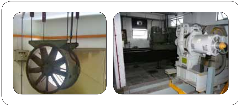
Figure 26: Examples of local ventilation system.
